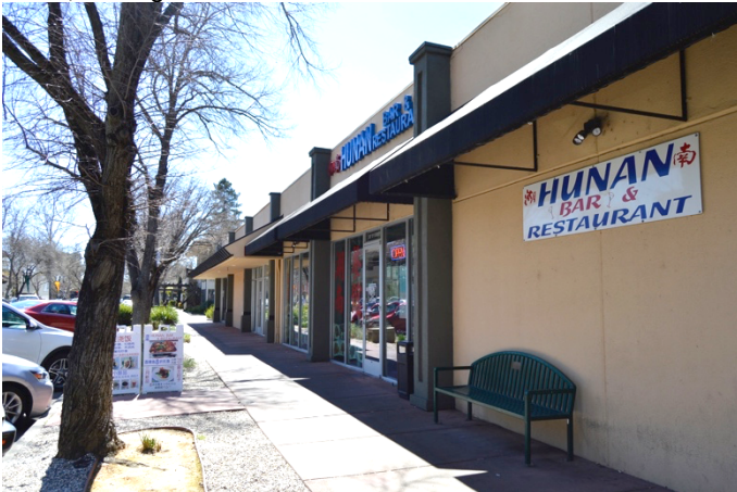
Figure 3. D Street storefronts, looking south.
